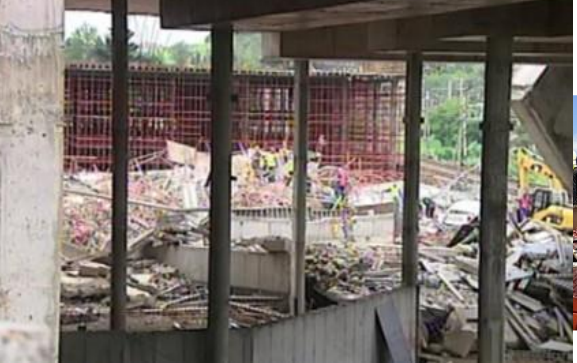
Tongaat Mall collapsed, killing two people and injuring 29 others.
